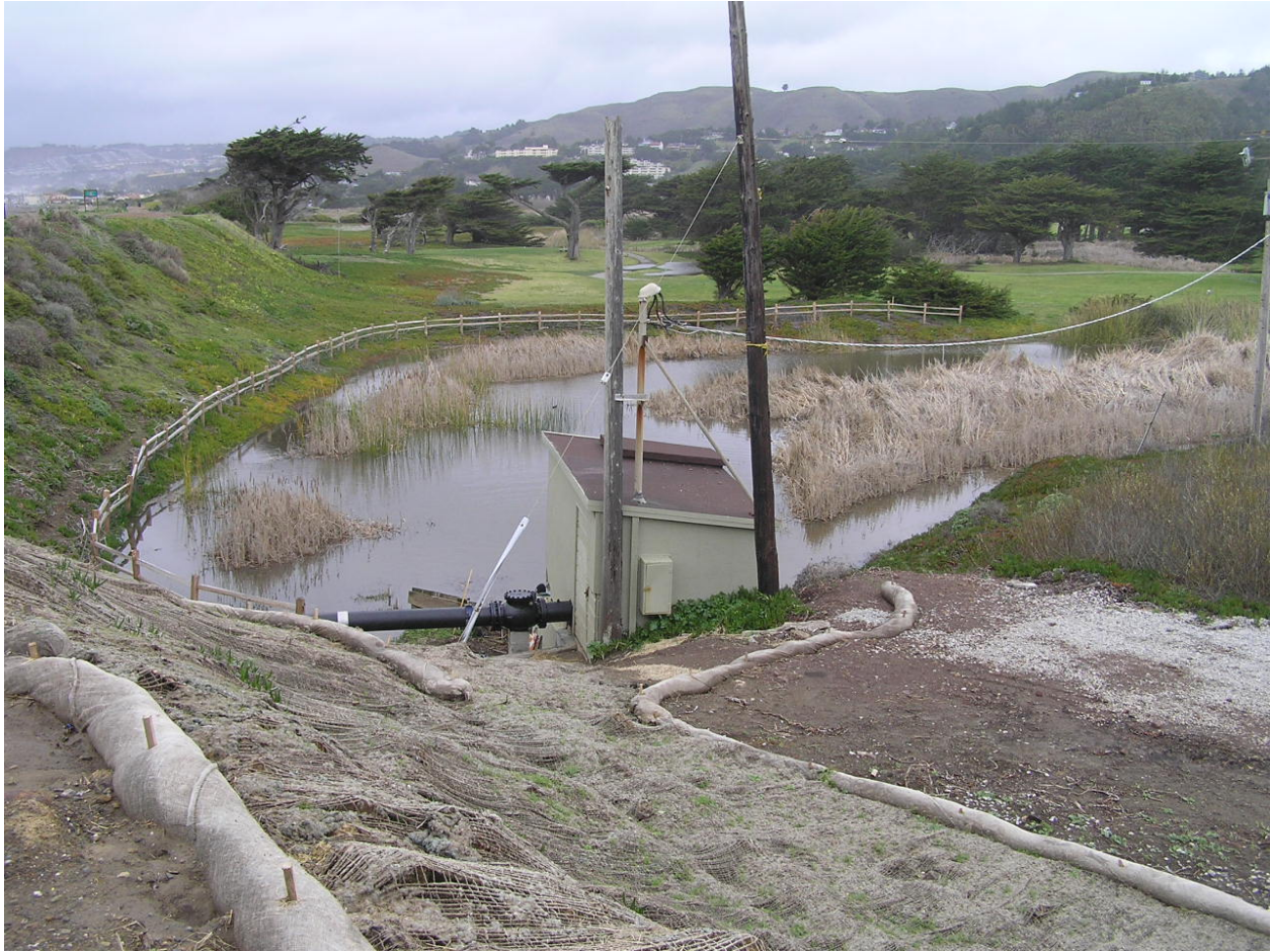
Figure 3. Artificially low maximum water levels of Laguna Salada. Horse Stable Pond at pump station, showing transient high lagoon surface elevations partially re-occupying artificially drained floodplains, February 17, 2009. Note partial flooding of fairways in background. Rapid drawdown due to pumping prevents seasonal wetland habitats from establishing in floodplain above tule marsh.
