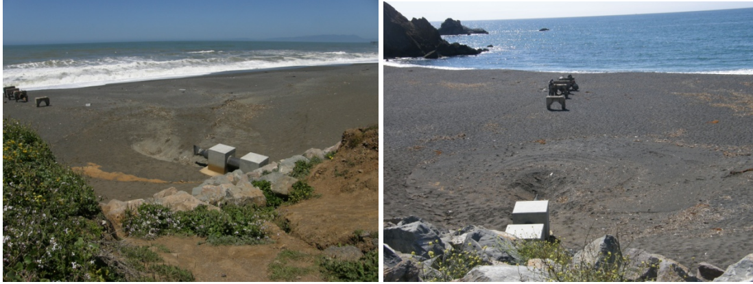
Figure 5. Drainage and discharge of Laguna Salada waters on Salada Beach during the dry season. The natural filling of Laguna Salada by Sanchez Creek low flows and groundwater discharges in summer is arrested by active pumping even in dry months, maintaining artificial drawdown of the lagoon to low levels all year. Discharge point below the outfall results in scour pools, internal drift-lines delineating high water levels in the pool, and an erosional discharge channel. Photo at left June 11, 2010. Right, August 17, 2010.
