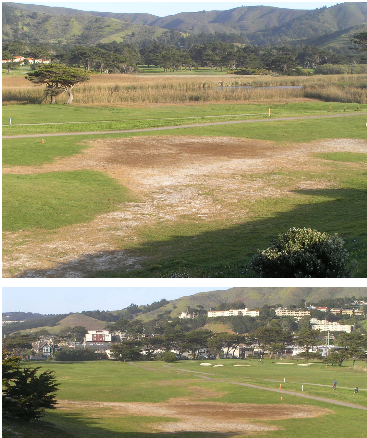
Figure F-1. Overview of saline seep patch in golf turf immediately behind levee at NW end of Sharp Park golf links appeared in February 2010 following high spring tides and high swell runup on adjacent beach, but no levee overtopping
